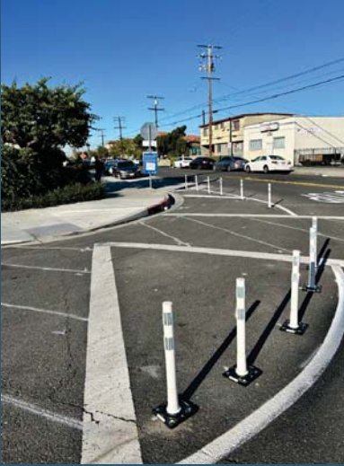
El Monte Quick-Build curb extension
