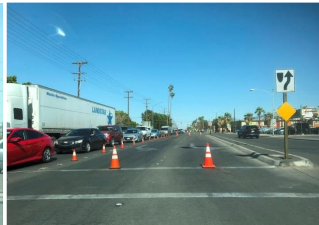
Left turn lane closure during peak hours on SR-98 at SR-111
