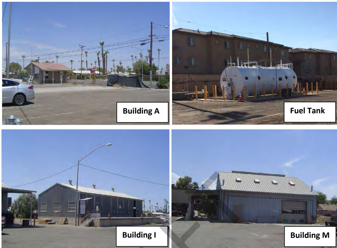
Figure 10-1. Existing Features To Be Demolished at Adams Avenue Site
