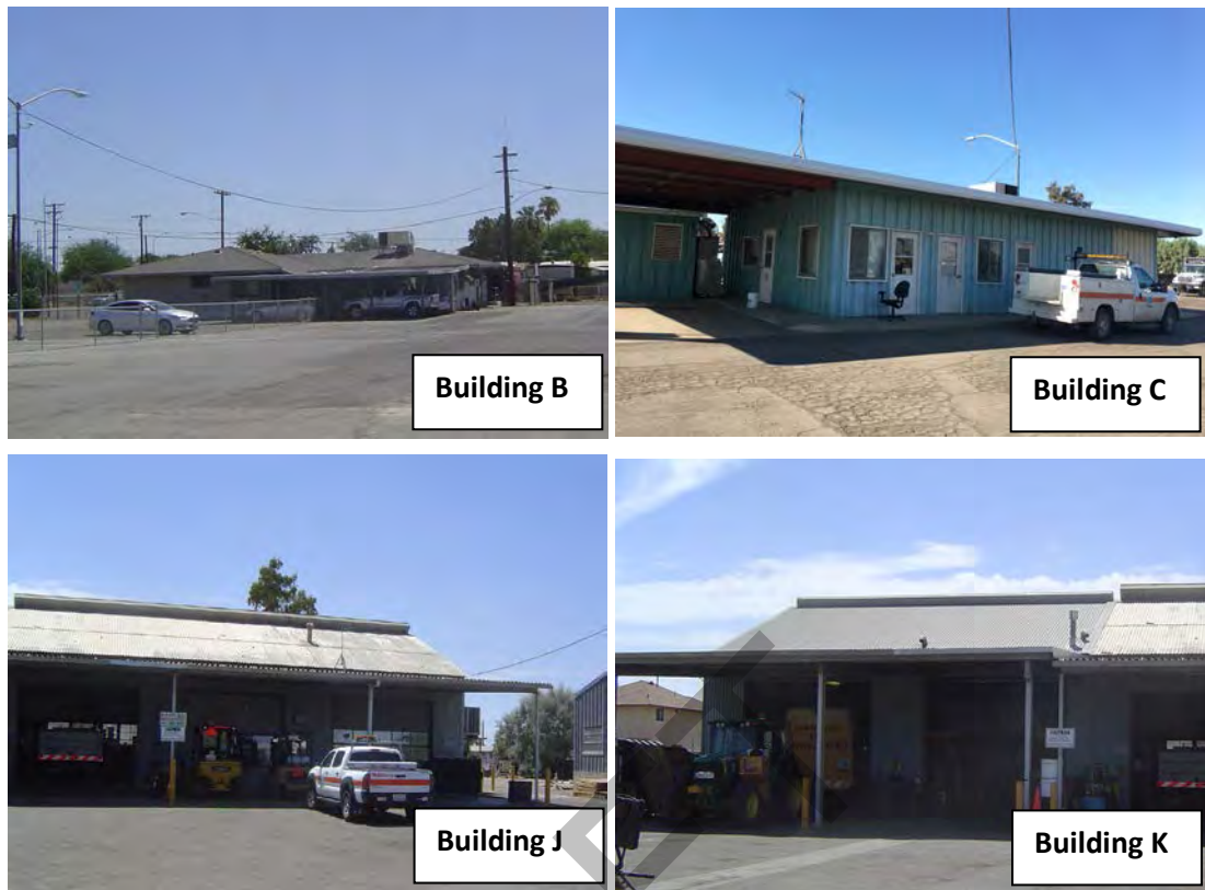
Figure 10-3. Existing Features To Be Kept at Adams Avenue Site
