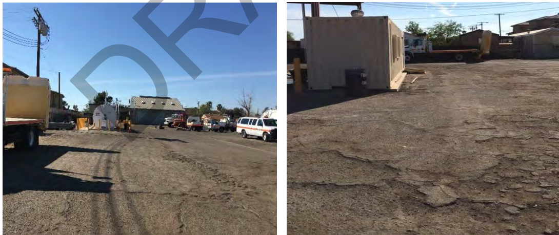
Figure 10-2. Existing Pavement Condition at Adams Avenue Site
